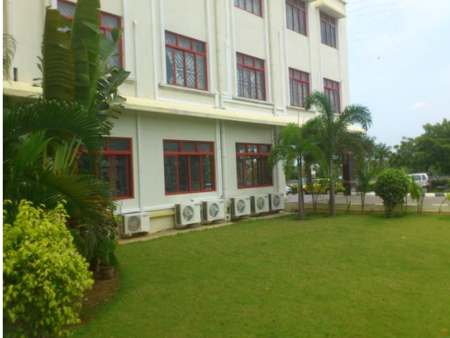
North Western side
